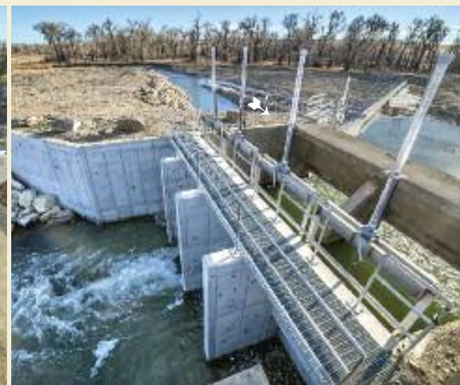
Renovated dam with rock ramp (arrow) for fish passage, February 2016.
