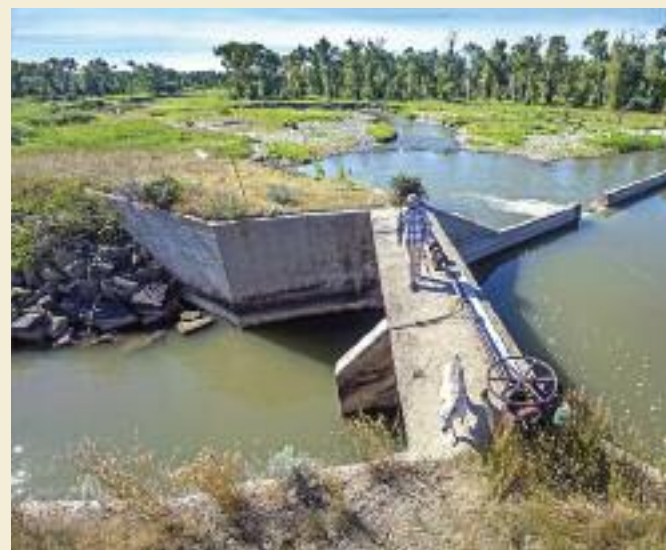
Deadman’s Reservoir Diversion Dam before reconstruction.
